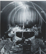
At the outfitting pier, near the tunnel site, concrete is added to interior and exterior portions of the tubes.
