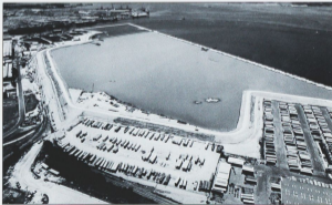
The 146-acre Canton/Seagirt Dredge Disposal Site will hold 3 1/2 million cubic yards of material dredged from the harbor bottom. It is anticipated that the site will be converted by others into a marine terminal in the future.
