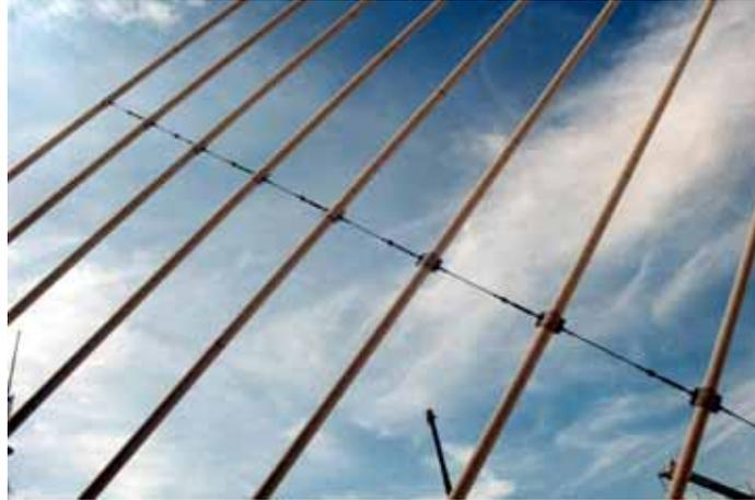
**Figure 11. Photo. Cable cross-tie system.**
