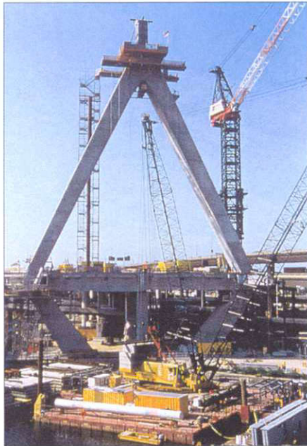
Fig. 4: Construction of north tower
