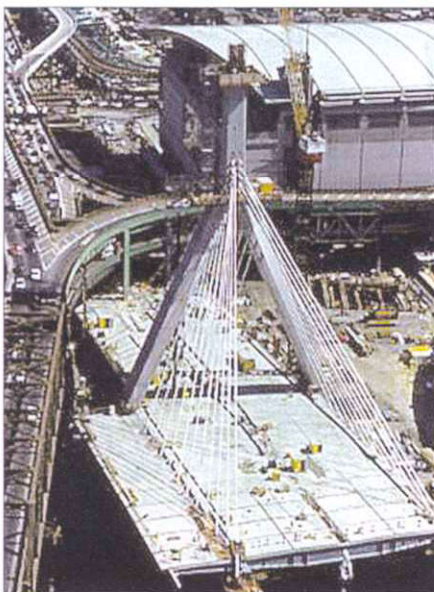
Fig. 2: Site constraints – The existing bridge (left) and subway tunnel (right)
