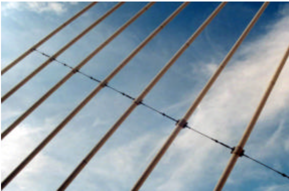
Figure 4: Cable Cross-ties
