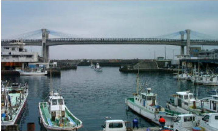
Figure 1: Odawara Blue Way Bridge, Japan (Photo by Takagi, Ryo)
